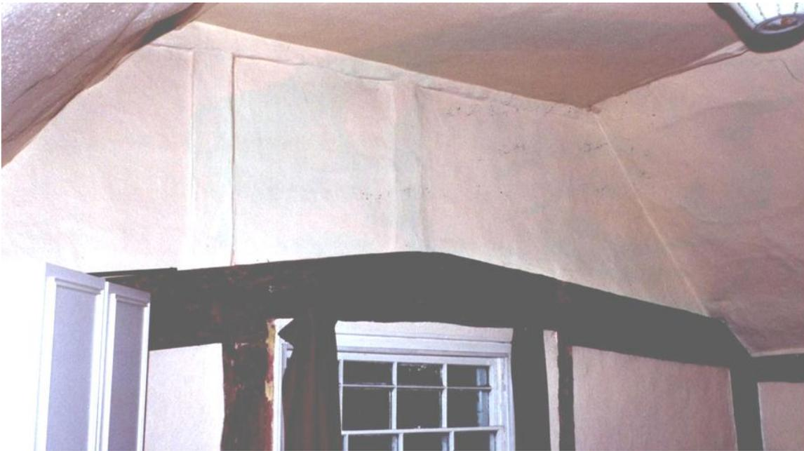
The opposite end with the North wing showing the roof of the wing of a trapped side purlin form, not so old as a Crown Post. Is there the shadow of a wind brace on the near roof pitch? (see the arrow)
