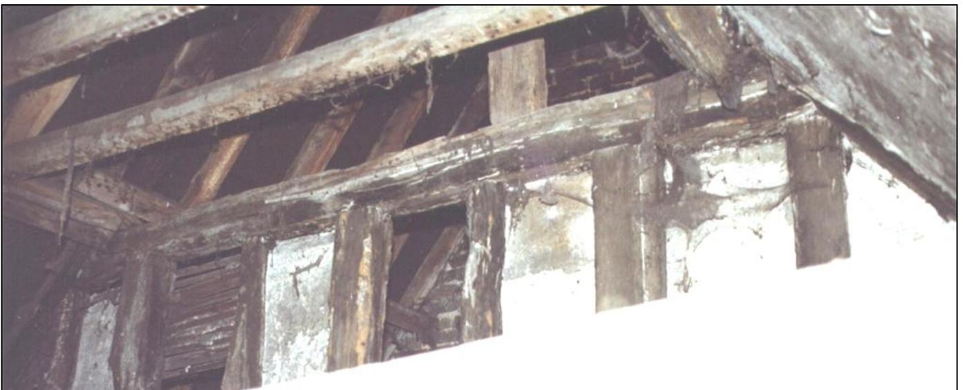
The timber-framed end of the North wing and beyond the end of the brick extension. (See p.13 for a plan of the building.)
